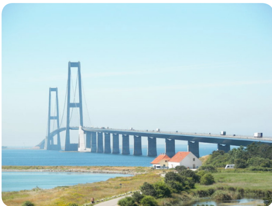
The Great Belt Bridge (Eastern part) - the second longest bridge in the world.
